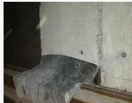
Peeling off EZY-NET® film after it has dried out, resulting in a clean surface.
